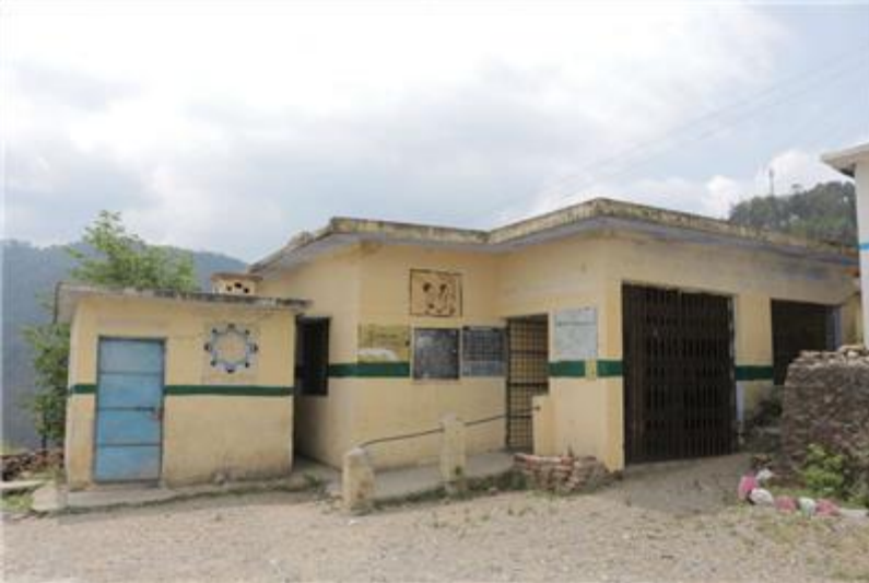
Exterior view of the school building where the new library is located.
