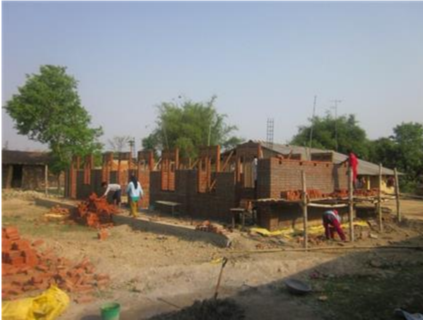
Ground floor wall construction work in progress.
